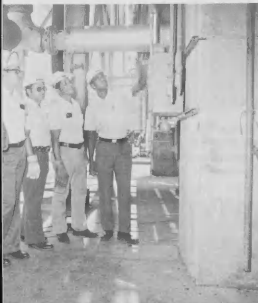
Adjusting the # 5 PS Crude furnace stack damper and observing the draft gauge reading are Eddy Laclé and R. Benjamin Lampe.
